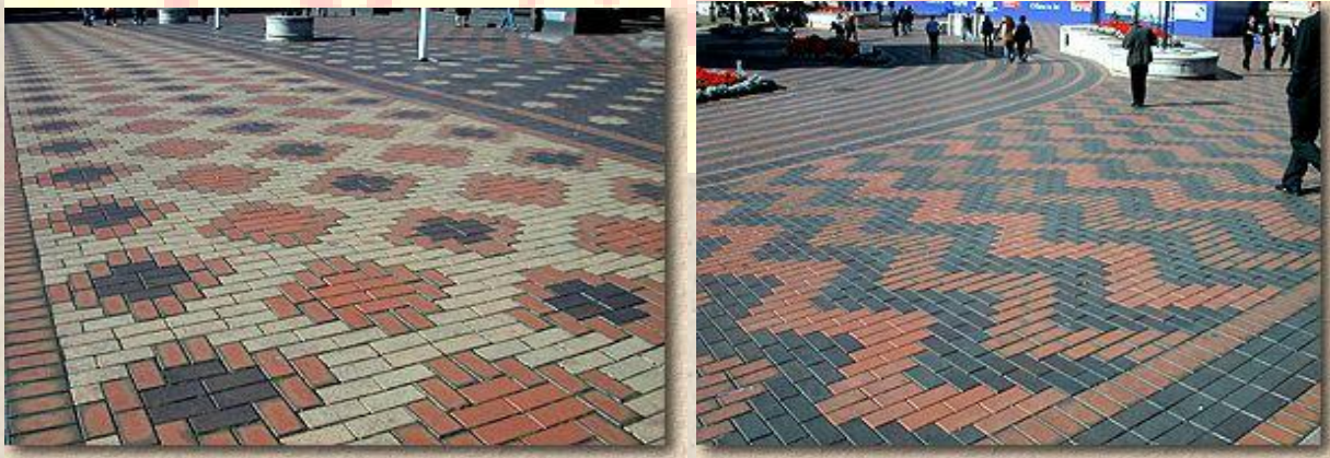
Newly completed clay pavers to private driveway
